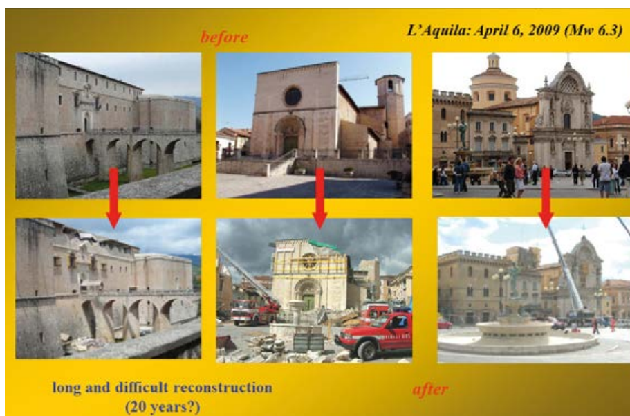
Figure 2: Heritage damage in L'Aquila after the 2009 seismic event.
