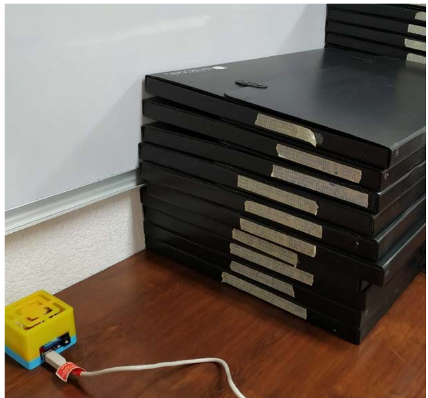
FIGURE 5. Installed Datalogger (Photograph: Gustavo Lozano, 2023).
