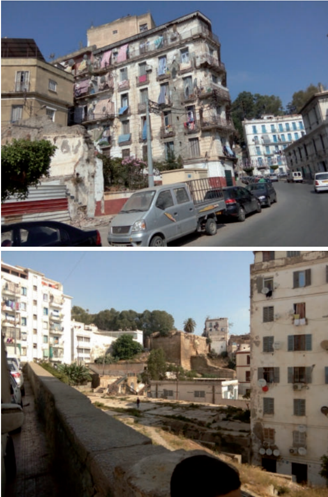
Figure 6.- Advanced state of degradation of the built environment in the south-west area Bellili district. Sr. author
