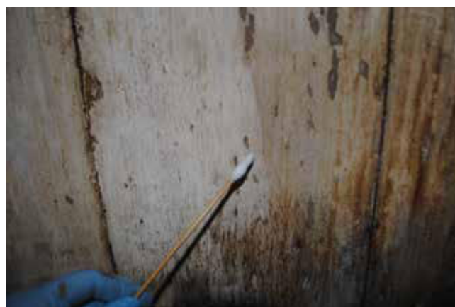
Figure 5.- Removal of the acrylic resin using both saturated and aromatic hydrocarbon solvents. Photographed by Patricia Monteiro.
