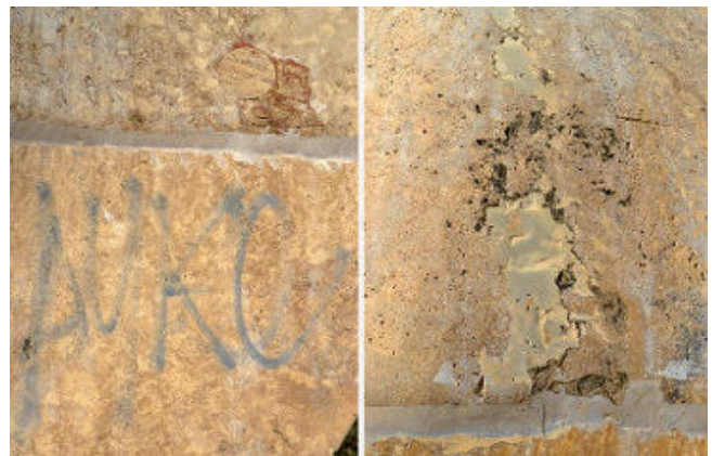
Figure 2.- Miguel Moreno, Luna . Natural stone, monumental proportions. Detail of the work's damage. Source: María del Carmen Bellido.
