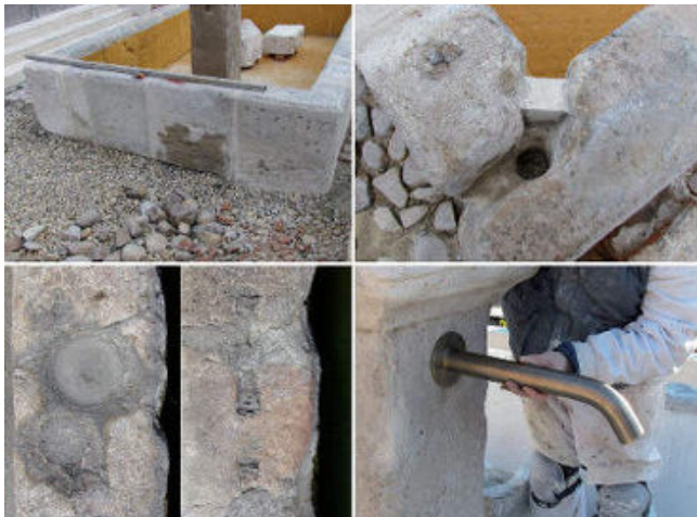
Figure 5.- Restoration details: substituting cement for limestone and pylon waterproofing; discovery of the primitive spillway corner; conservation and protection of the original remains; new sewers made of brass as per the primal design.
